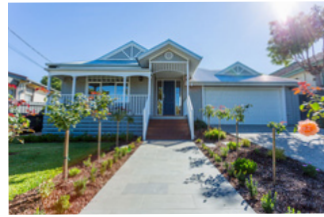
Mornington House $2,450 m 2
