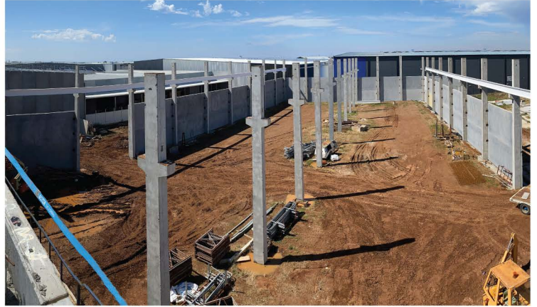
Factory structure as seen from the office roof.
