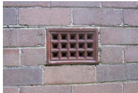
An example of what a sub-floor ventilator may look like.
